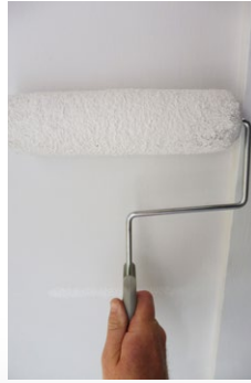
Step seven Roll the remainder of the ceiling and allow two hours for paint to dry.
