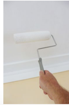
Step eight Repeat steps six and seven and allow the ceiling paint to dry.
