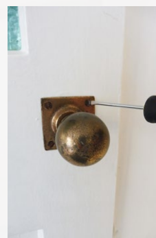
Step sixteen Carefully replace door handles and light switch and socket cover plates.
