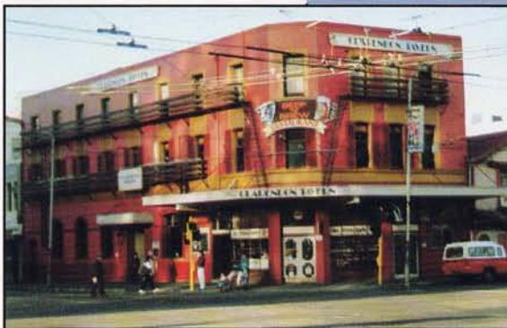
Pictured here in startling contrast is the transformation from the old Clarendon Hotel to the new Glass House.
