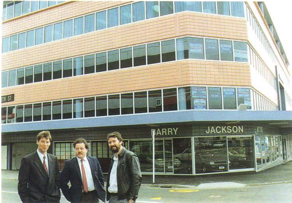
Resene Paints Limited Architectural representative Nicholas Nightingale with Bruce Dunnet of New Zealand Protective Coatings, the Contractor, who applied Uracryl, and Steve Grant of Comesky Grant, Architects.
