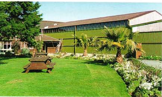
As green as grass - a section of the rest of the Matua Valley complex.
