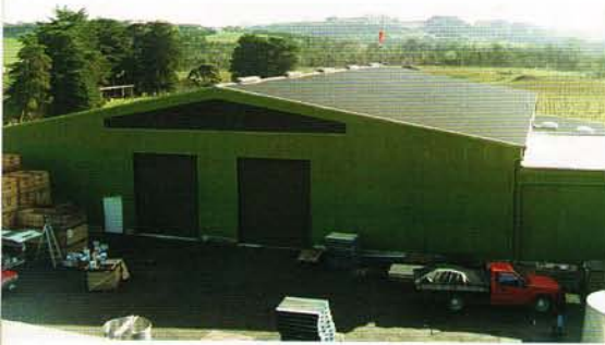
An end view of the new Matua Valley warehouse.
