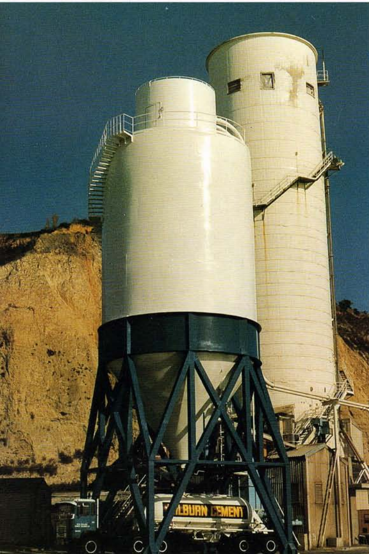
Ameron-treated Napier silos (above) and top right, Don Campbell with the Thorndon silos.
