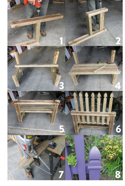
Screw 2 x 400mm lengths and 1 x 800mm length together with the 75mm screws, as shown, to form the seat and leg frame.
