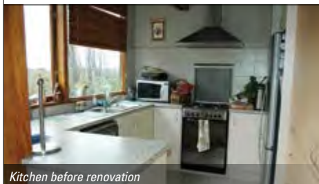
Kitchen before renovation
