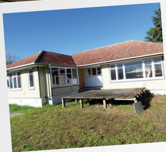
BEFORE: The ex-gang house was purchased for $92,000 and the total cost of renovating was $105,000.
